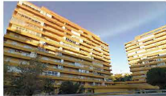
SPAIN-Staff Dormitory, Spain
