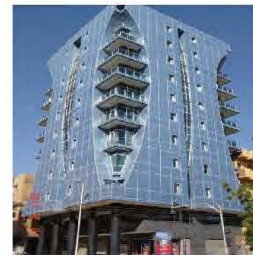
Sudan-Office Building, Sudan
